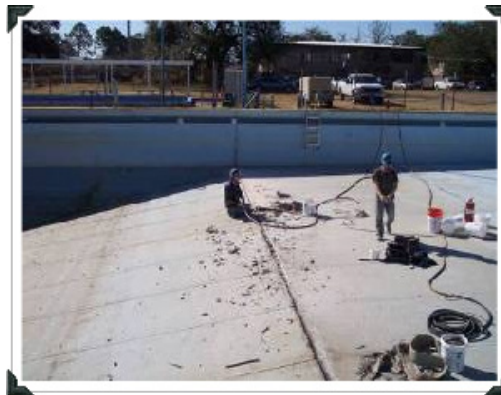
Pictured left and below: Expansion joint upgrades
