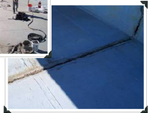
Pictured left and below: Expansion joint upgrades
