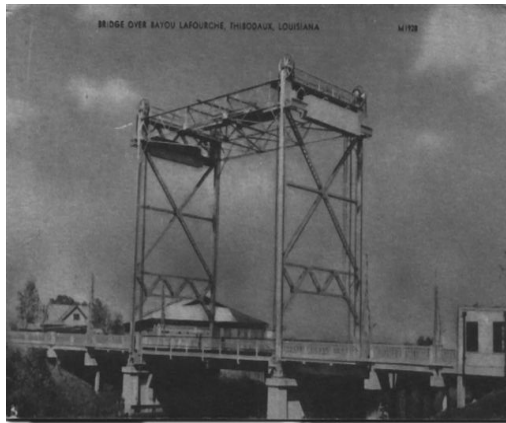
Bridge Over Bayou Lafourche, Thibodaux, La.
