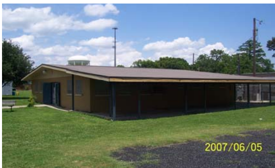
MLK Recreation Center Before Renovation.
